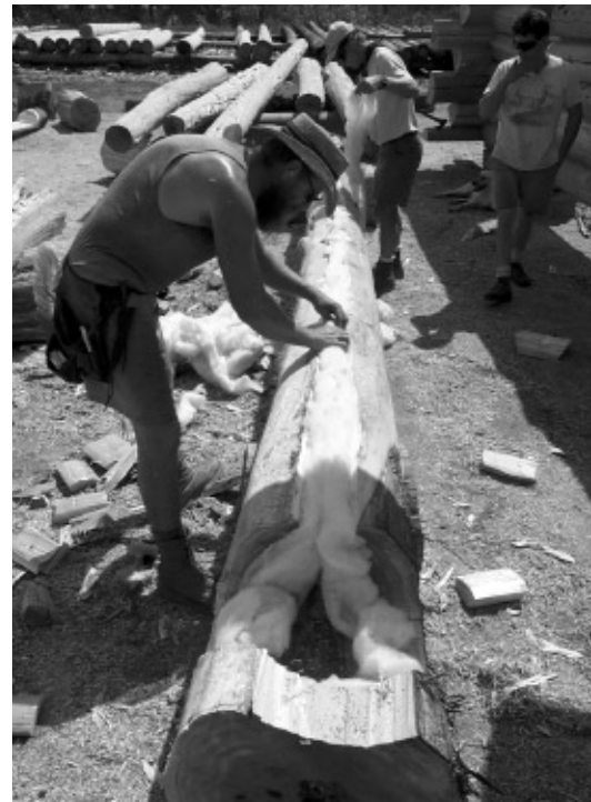
Wool being fitted into a lateral groove.
