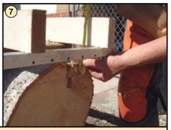
Measure down from the top of the 2 x 4 and determine the location of your first cut. If your log tapers you will be cutting a thicker slab at the large end of the log. Try to cut the smallest possible slab on this first cut. Make sure you lower the mill enough to miss whatever toe nailing you may have done.
