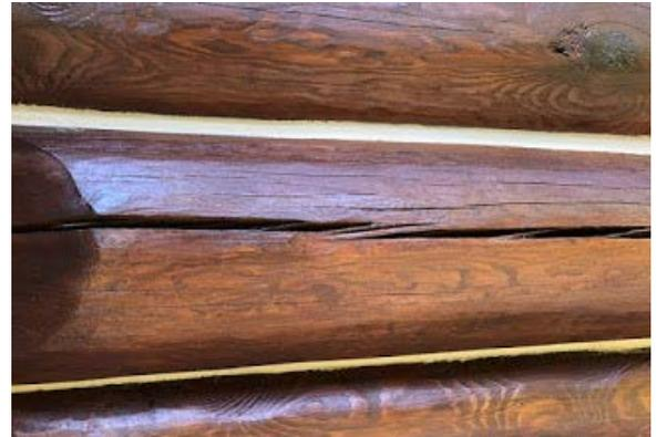
ing. Besides the appearance there are some things that need to be addressed when checks are on the exterior of a structure. Foremost, upward facing checks are like gutters, collecting water in all its forms. This water becomes trapped and is absorbed in the wood fibers. It then starts to decay the wood internally where it can not be seen. Even if the logs look fine on the exterior, stain and sealers are doing their job. The hidden damages can cause expensive log replacement.
