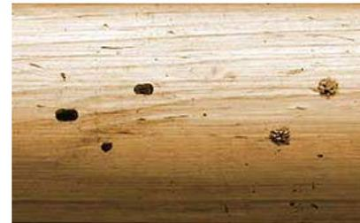
**To Avoid:** Fill any existing beetle holes with a quality [caulk](#) or [chinking](#).
