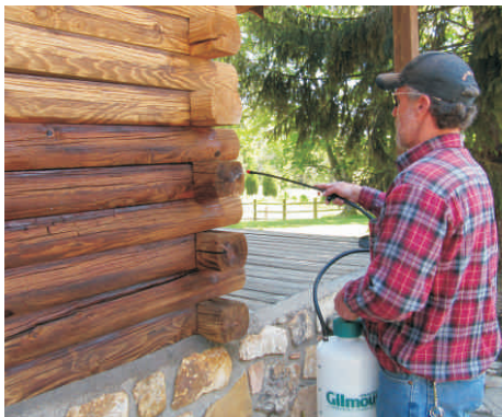
Applying a borate solution
