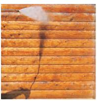
Step 8: Once the entire wall is pressure washed, rinse the wall starting at the top and work down. At this stage water volume is more important than pressure.
